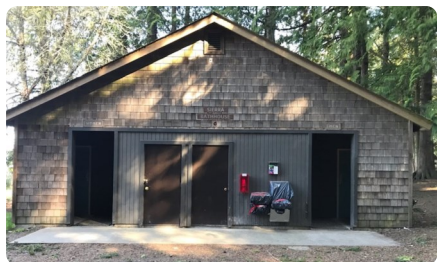
Main Camp Bathrooms & Showerhouses
